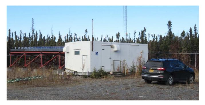
Figure 3 ~ MUIR equipment enclosure and associated radar antenna array (left-background). All electronics for the Callisto-LWA Antenna installation were placed in the enclosure at the end of September. A protected coaxial cable entrance facility was installed on the back of the enclosure (not visible in this picture). This picture was taken the day before the weather station and lightning sensor was installed on the enclosure. Image © 2021 W. Reeve
