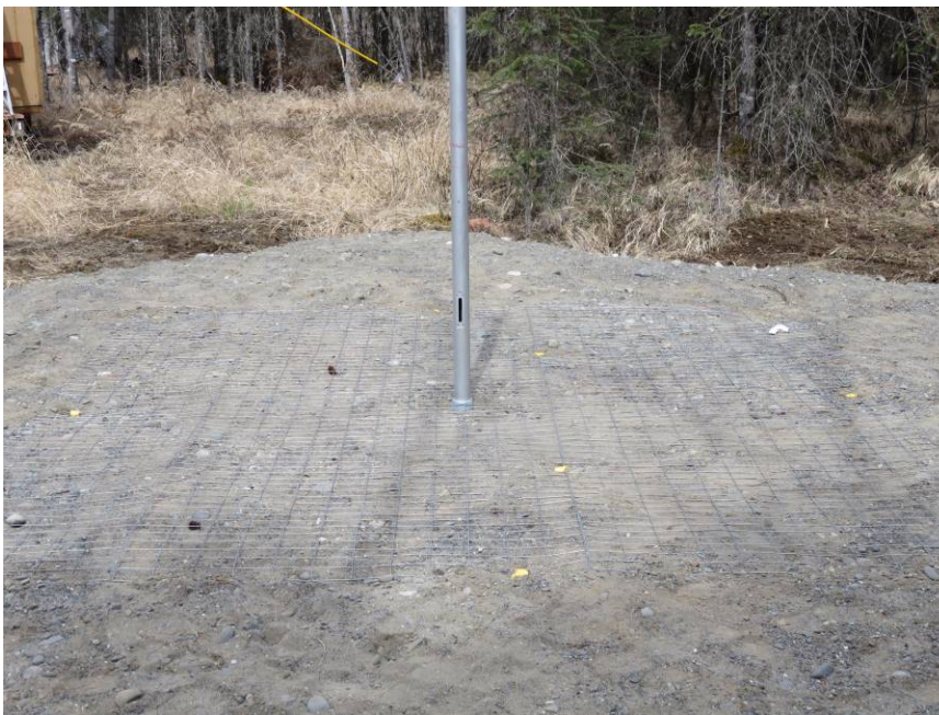
Figure 5 ~ After the stake and mast were installed, the 10 x 10 ft (3 x 3 m) ground grid was placed on the pad and centered on the mast. The mesh is oriented north-south and east-west, the same as the dipoles. It is held down in several places with yellow plastic tent stakes. Note the milled slot (black line) in the lower part of the mast. A modified type E PVC conduit fitting is attached later over the slot and the coaxial cables are then fed up through the conduit fitting into the mast and up to the FEE located at the top. Image © 2017 W. Reeve
