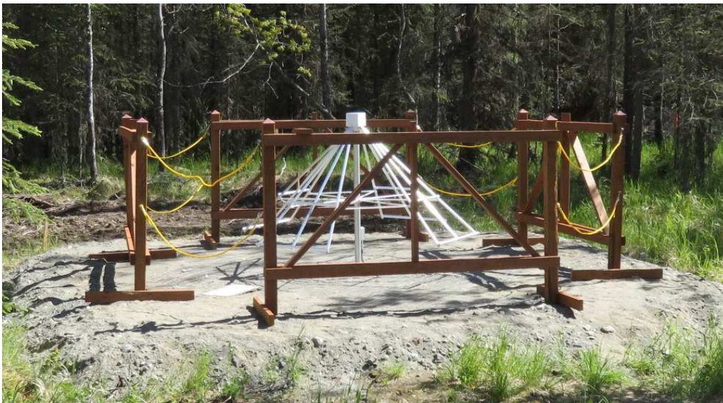
Figure 1 ~ LWA antenna installed at Cohoe Radio Observatory during May and June 2017. This single antenna is used for studying solar radio emissions and HF and low VHF propagation. The antenna is built on a gravel pad and protected from marauding moose by a simple wood barrier. Image © 2017 W. Reeve
