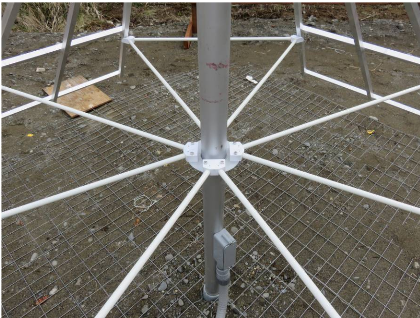
Figure 19 ~ View of the support flange and fiberglass frames. The bottom of the flange (not visible) has set screws for securing it to the mast after the link and tie rod frame assemblies are set at the proper height and are level; when all parts are properly assembled the tie and link rods are perfectly horizontal. Image © 2017 W. Reeve
