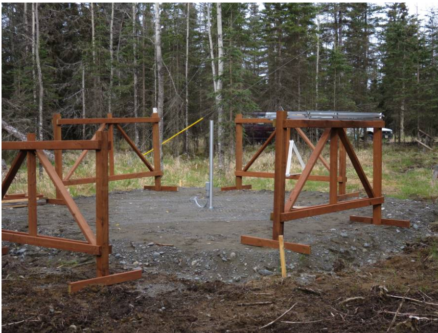
Figure 11 ~ The moose fence was built in four sections, three of which are placed close to final position on the pad in this image. The fourth section at left is ready to be moved onto the pad. I originally planned to use ground stakes for the fence posts but later decided to make the fence sections easily movable by fastening them to cross-braces. The fence uses only enough material to prevent moose from getting close to the antenna and hopefully not significantly disturbing the antenna pattern. The only metal used in the fence is in the screws used to hold the pieces together. These screws are compatible with the chemicals used in the wood treatment. Image © 2017 W. Reeve
