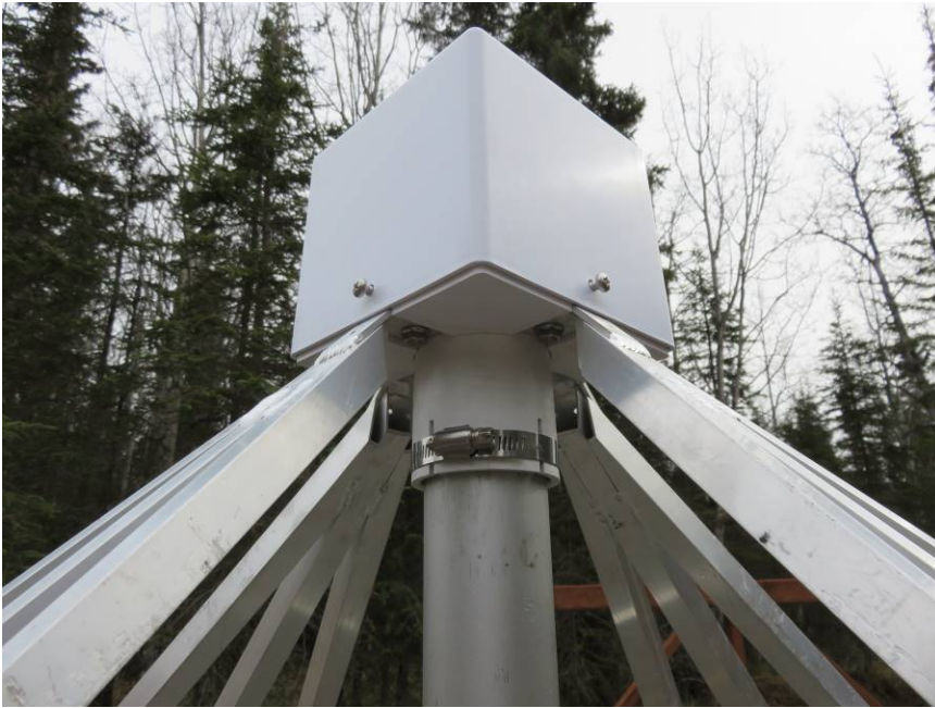
Figure 22 ~Closeup view of the FEE enclosure cover and hub baseplate. The bottom of the baseplate has a tube with four slits. The tube is slipped over the mast and a stainless-steel worm-gear clamp is installed that squeezes the tube for a tight fit. The antenna elements are fastened underneath the baseplate to threaded studs using flange nuts. Image © 2017 W. Reeve
