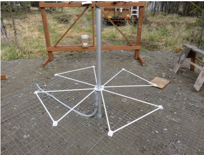
Figure 13 ~ The completed flange and fiberglass frame assembly has been slipped over the mast and is resting on the conduit fitting. By this time the excess coaxial cable has been pulled back to top of mast. Image © 2017 W. Reeve
