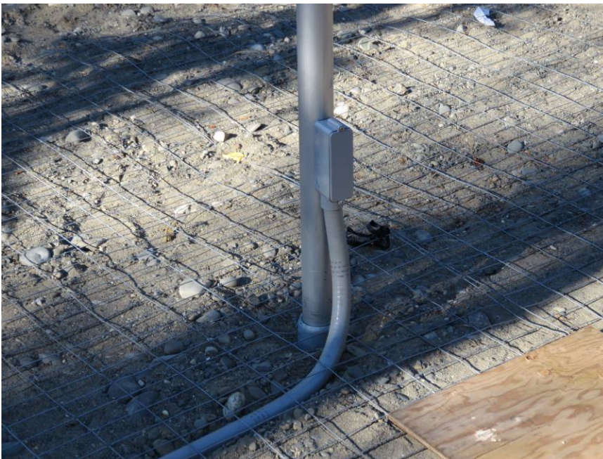
Figure 9 ~ Conduit installation detail. As mentioned above, the mast is milled to accept the modified conduit fitting supplied with the antenna. The fitting is fastened to the mast with two screws. In most installations the conduit is simply slipped up into the conduit fitting without a conduit connector, but I later installed a connector to reduce movement of the conduit during the freeze-thaw cycles at this sub-arctic location. In many installations, only a short piece of conduit is used to protect the coaxial cables from rodents and the cables are direct-buried. Image © 2017 W. Reeve
