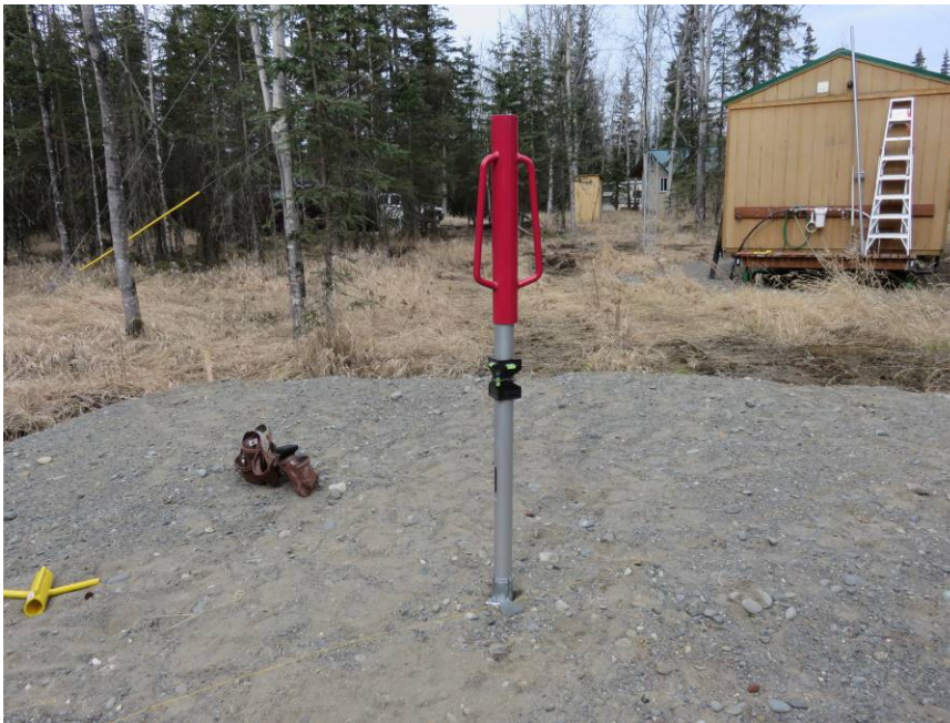
Figure 4 ~ The first order of business in May 2017 was to locate the center of the pad and drive the galvanized steel OZ-Post ground stake that supports the antenna mast. The stake was hand-driven with a weighted driver – the red tubular structure with handles on top of the mast. The stake penetrates the ground about 28 in (0.9 m) and provides a very stiff foundation. The mast was held vertical during the driving operation with the aid of a post level strapped to the mast just below the driver. A collar clamps the mast in position on the stake collet. The collar can be seated with a heavy hammer and a wood block but I used the yellow purpose-built tool on the ground in the left foreground of the image. Image © 2017 W. Reeve
