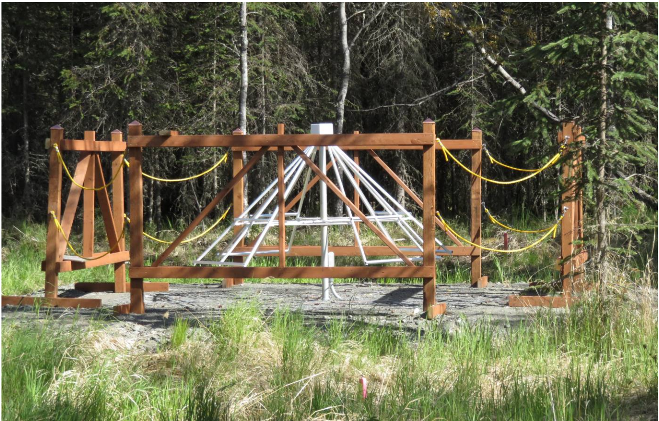
Figure 28 ~ Completed antenna installation and moose fence. The four fence sections are connected with loose 1/2 in polypropylene ropes with clips that attach to threaded eyes on the fence posts. The removable ropes allow easy access for maintenance but prevent moose from entering the space around the antenna. This image was taken on 1 June 2017 as the surrounding foliage was turning green for the summer. Image © 2017 W. Reeve
