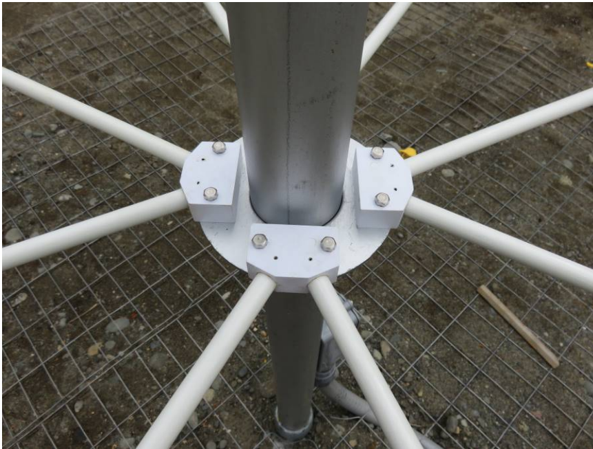
Figure 20 ~ Closeup view of the fiberglass frame support flange. All fasteners are stainless-steel; the ones shown here that hold the trapezoidal blocks to the flange are 10-32 hex head machine screws. Also visible here are the small holes in the blocks for pins that secure the fiberglass rods to the blocks. Image © 2017 W. Reeve
