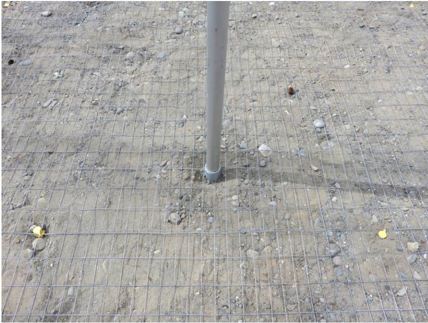
Figure 6 ~ Ground grid details. The grid is made from 4 ft (1.2 m) wide rolls of 14 AWG (2 mm) galvanized welded steel garden fence mesh. To obtain the required overall dimensions, three overlapping sections were joined with swaged Nicopress splicing sleeves. The wires were cut in the center of the grid to accommodate the mast. Two yellow tent stakes, which hold the grid down, are visible in the left and right foreground. The grid does not need to be bonded to the mast. Image © 2017 W. Reeve
