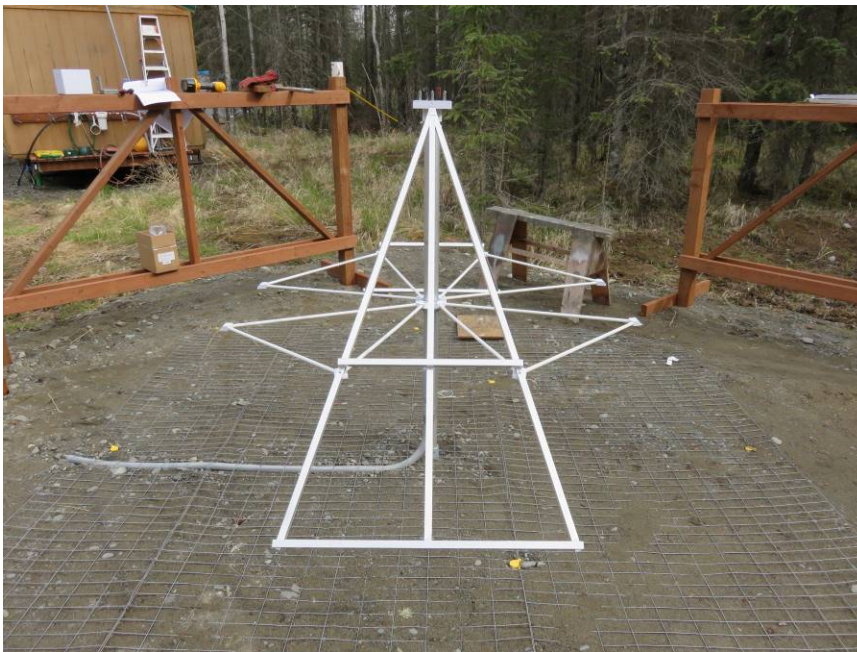
Figure 15 ~View looking north shows the first pair of dipole elements that have been placed and oriented. Before the clamp on the top hub and the fasteners on the support frame flange and elements are tightened, the elements are rotated to the desired direction and the fiberglass triangular frames are leveled. In the LWA, all antennas are referenced to true north (dipole elements are oriented north-south and east-west). In single antenna applications specific orientation is not necessary; however, at CRO, the antenna is referenced to true north in case I decide to install additional antennas for a future array. Image © 2017 W. Reeve
