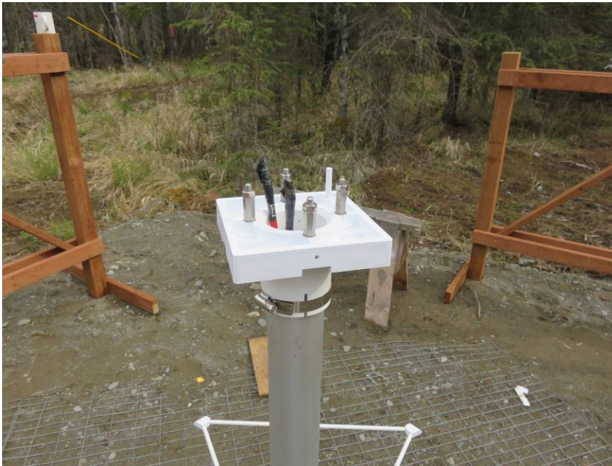
Figure 14 ~ FEE hub baseplate installed on the mast. The clamp at the base of the hub has not been tightened. Note the two coaxial cables have been taped to keep moisture out. Prior to being pulled through the conduit, the cables were marked at both ends with green and red colored tape for identification. Image © 2017 W. Reeve
