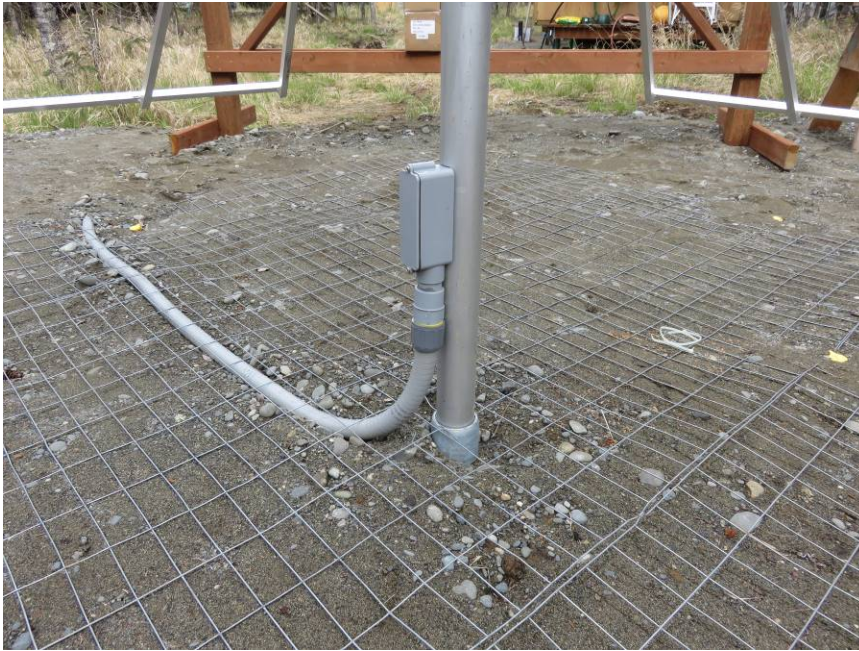
Figure 24 ~ View of the type E conduit fitting, conduit and conduit connector. The conduit connector was installed after the conduit installation. The conduit connector is not necessary in most installations and is not supplied with the antenna. The cover on the conduit fitting has a rubber gasket to keep moisture out. Image © 2017 W. Reeve
