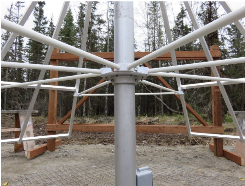
Figure 21 ~ Closeup view of underside of the center flange. Two of the four hex set screws that hold the flange in place on the mast are visible. The antenna assembly is very rigid and will survive 90 mph ( 145 \text{ km h}^{-1} ) winds. Winds that high never occur at Coho but have at other antenna installations around the world. Image © 2017 W. Reeve
