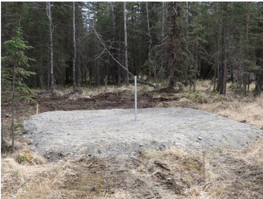
Figure 7 ~ Pad, mast (center of image) and ground grid ready for installation of transmission lines and remaining antenna components. This image was taken on 7 May 2017 before the ground cover and deciduous trees turned green. The antenna is 40 ft (12 m) from the observatory building. Image © 2017 W. Reeve
