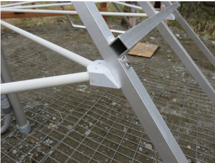
Figure 23 ~ Closeup view of fiberglass support block for the aluminum elements. A single 10-32 hex head stainless-steel machine screw on each side of the dipole element frame holds the frame to the block. Image © 2017 W. Reeve
