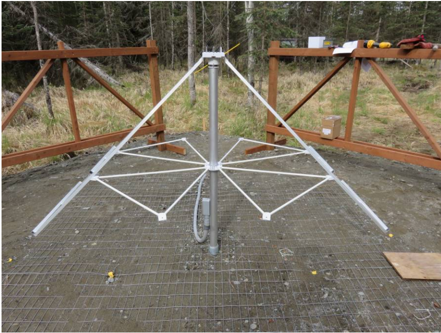
Figure 16 ~ Another view of the north-south dipole. This view is looking west. The elements of each dipole form a right angle at their vertex. During assembly the fasteners are not fully tightened until all the components have been placed and aligned. Image © 2017 W. Reeve
