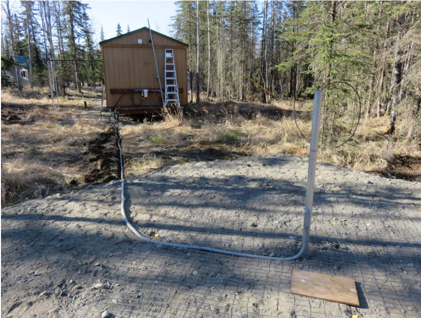
Figure 8 ~ Liquid-tight, flexible, non-metallic conduit was installed below the ground grid and in a shallow trench to the observatory building seen in the background. The conduit is 1 in trade size and 50 ft (15 m) long. It ends under the left side of the building. Before backfilling the trench, two LMR-240 coaxial cables (6 mm diameter) were pulled through the conduit; excess lengths of cable are barely visible hanging over the top of the mast. SMA-M connectors at the FEE end were installed before the cables were pulled through the conduit. The observatory ends were connectorized later. Image © 2017 W. Reeve
