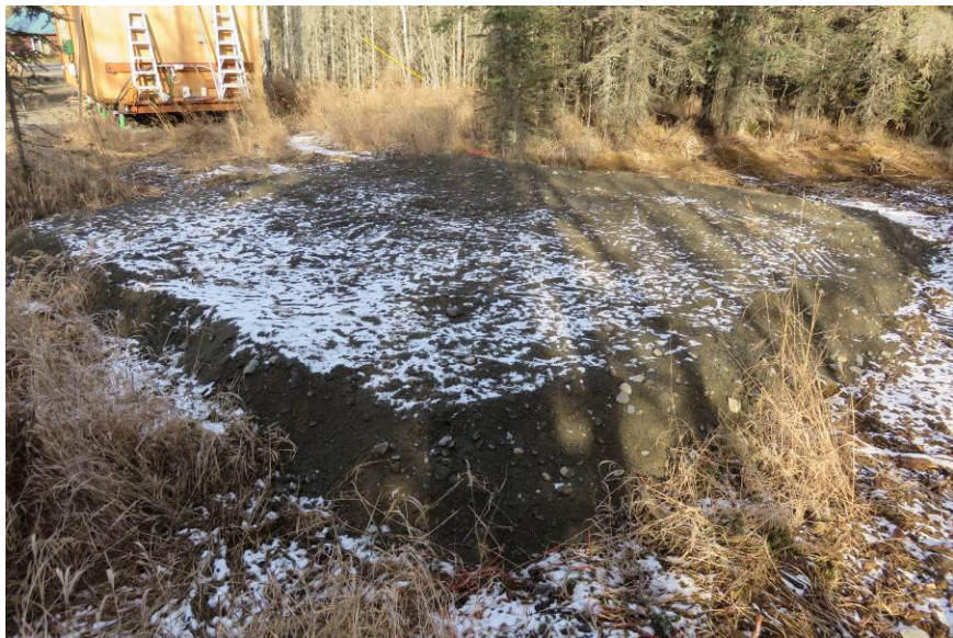
Figure 3 ~ A 25 x 25 ft (8 x 8 m) gravel pad was built for the LWA antenna. It has a light dusting of snow soon after being finished in mid-October 2016. The pad location and corners were staked and an excavator was used to remove the peat and clay overburden and tree roots from the pad area to a depth of about 4 ft (1.2 m) – down to the underlying glacial moraine gravel from the last Ice Age. Next, the area to the right of the image was excavated to mine the gravel for the pad. Finally, the pit excavated during the mining was backfilled with the debris and leveled. The pad was left to settle over the winter until May 2017. Image © 2016 W. Reeve
