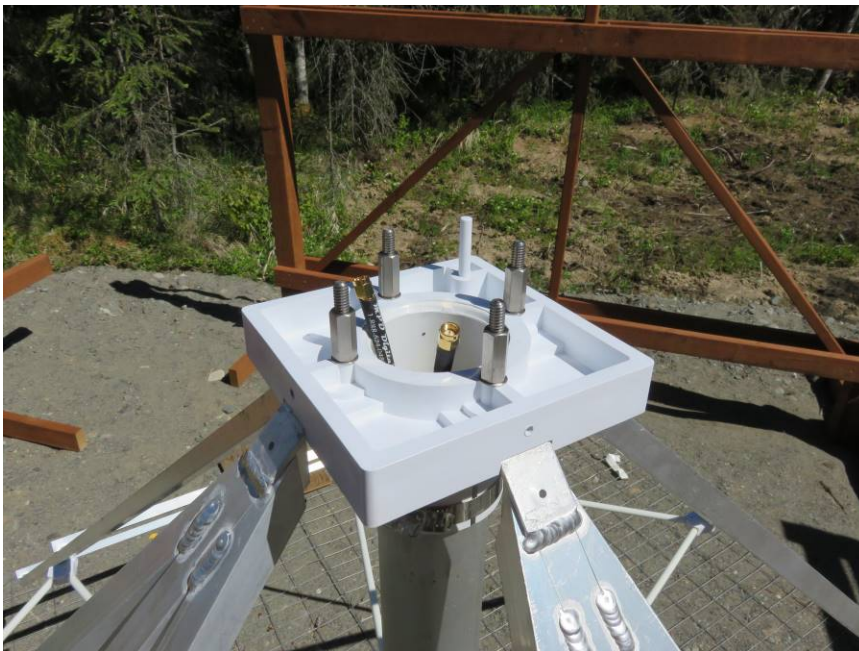
Figure 25 ~ The cover has been removed from the FEE hub baseplate. Note the FEE alignment pin in the back corner of the baseplate. This view also shows the four 1/4 in coupling nuts and studs that hold the FEE PCB assembly in place and also connect the FEE to the dipole elements. Each element is fastened to a 1/4 in stud underneath the baseplate. The two coaxial cables are visible and the protective tape has been removed to ready them for connection to the FEE. This view also shows some of the aluminum welds in the foreground. Image © 2017 W. Reeve
