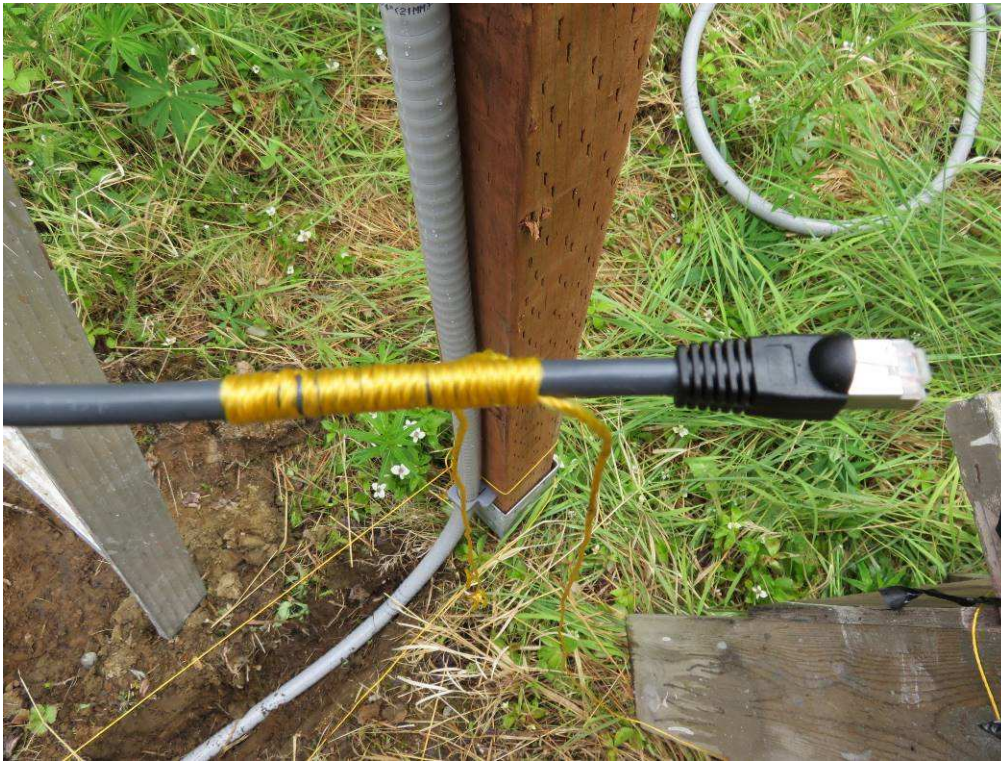
Figure 9 ~ Cable preparation for pulling.
