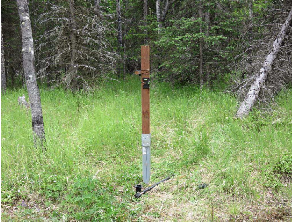
Figure 6 ~ Preparation for driving the galvanized steel post anchor.
