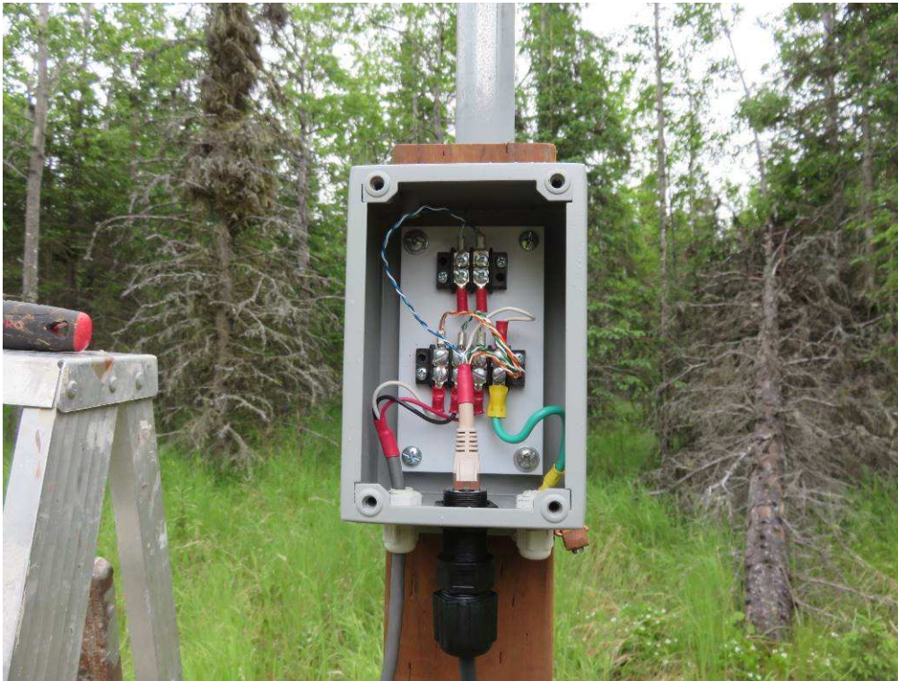
Figure 10 ~ Antenna junction box
