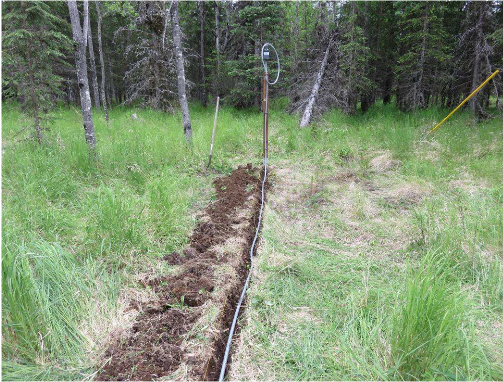
Figure 8 ~ Flexible conduit installation.
