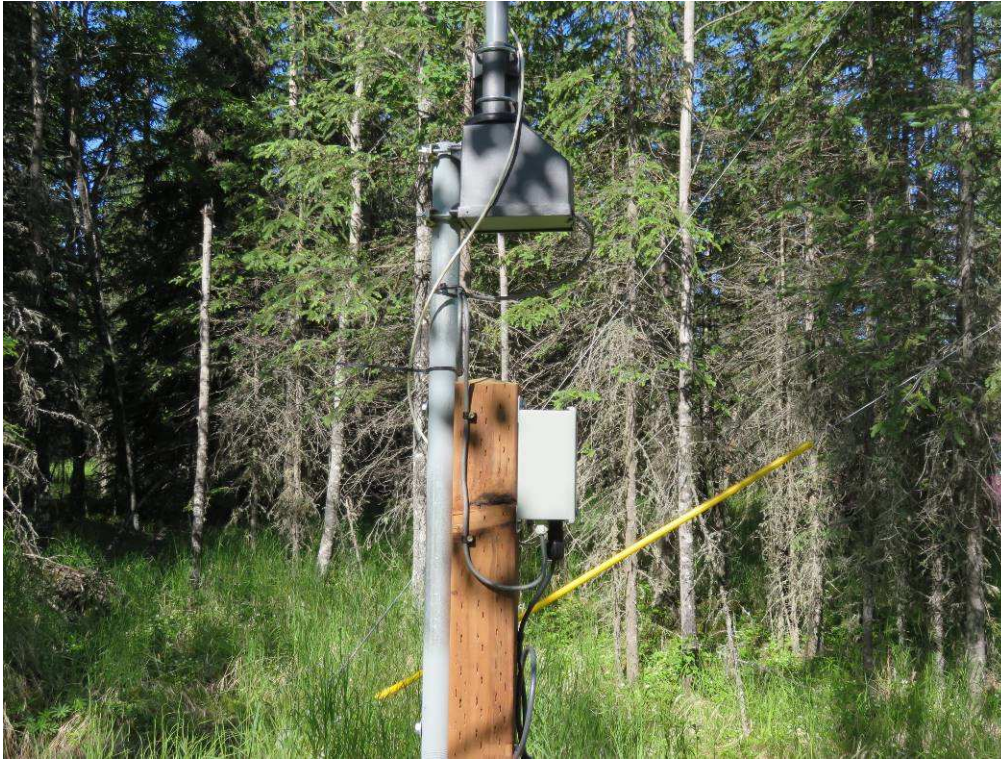
Figure 11 ~ Rotator and antenna junction box.
