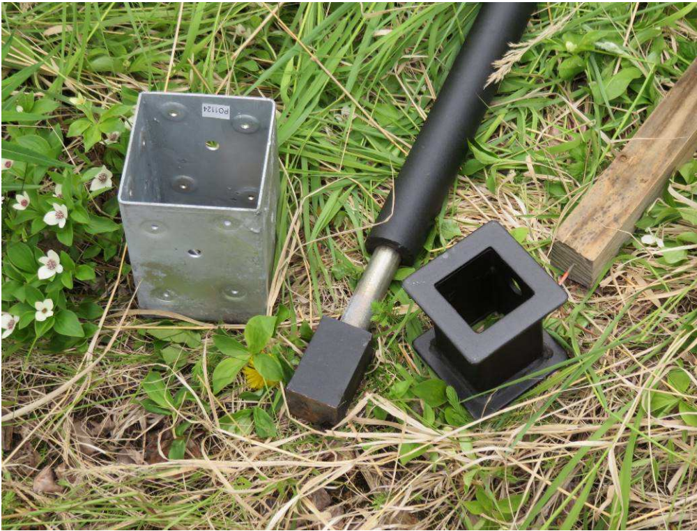
Figure 7 ~ Anchor and wood post installation, completed.
