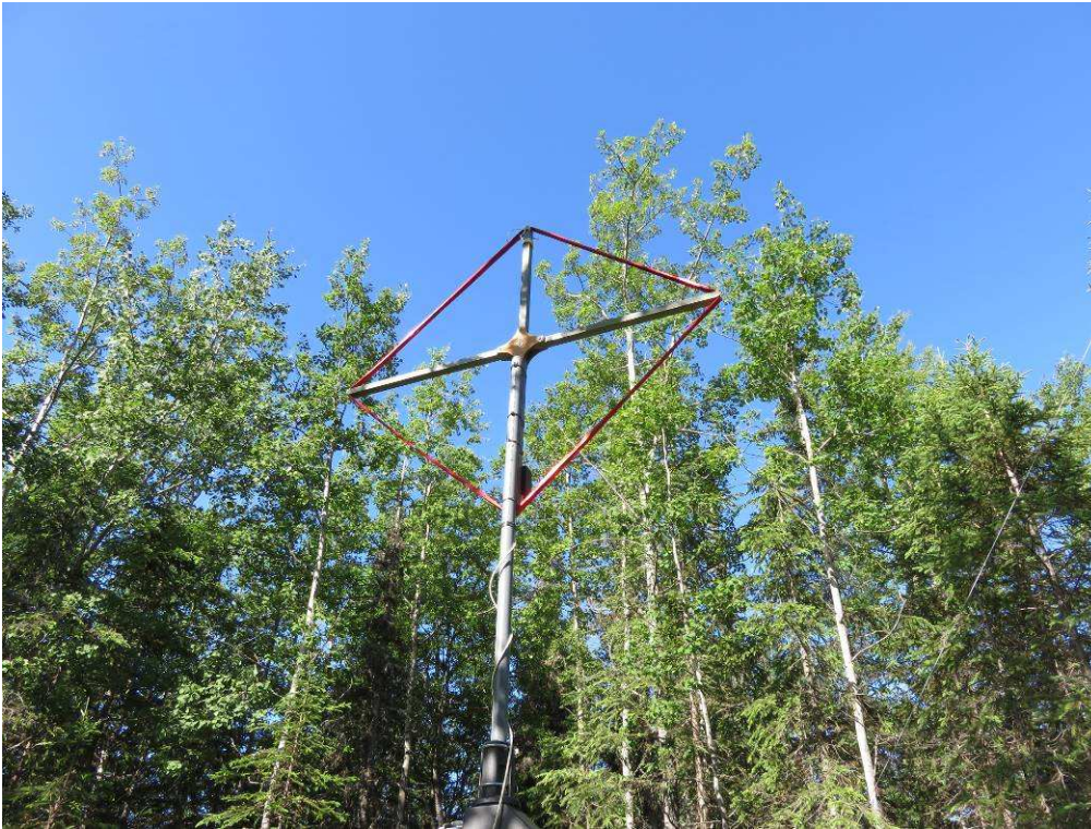
Figure 13 ~ Completed loop antenna installation ready for service.
