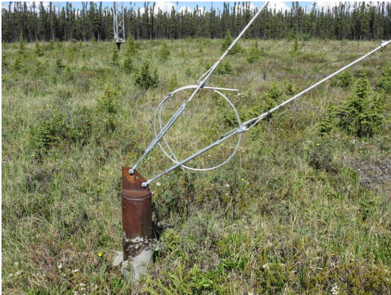
Figure 3 ~ Typical guy anchor consists of a steel piling capped with a bracket for fastening the guy strand turnbuckles. The piling is wrapped with polyethylene sheeting that provides a sliding surface to prevent frost jacking. The base of one tower is seen in the upper-left-background. It uses a similar piling except the top is capped with a 1 in thick steel plate on which the tower is placed. Image © 2019 W. Reeve
