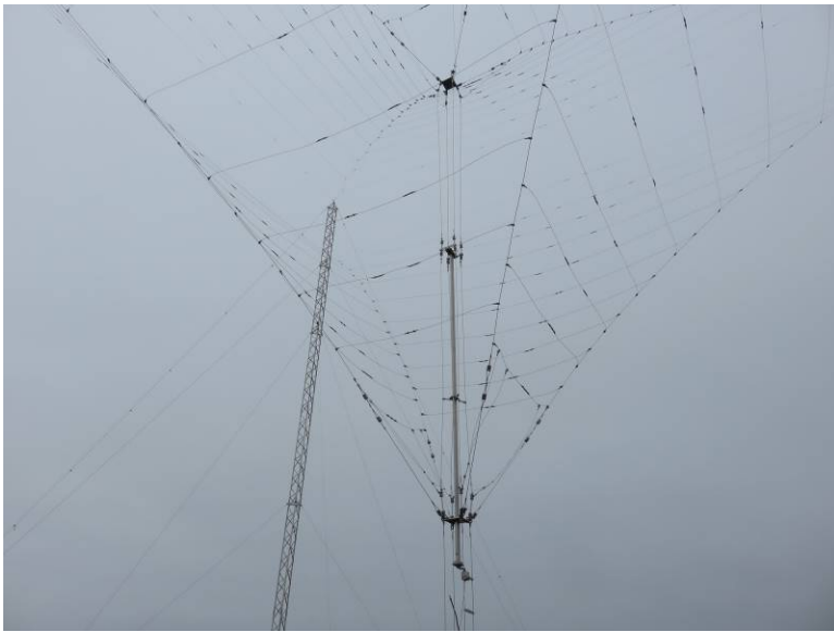
Figure 4.b (left) ~ Image from the ground of some of the stacked antenna wire elements for the lower cone and the impedance matching structure. The elements couple to the impedance matching structure in the middle. The balun is at the base of the structure; see text. One of four towers is in the left-background. Image © 2019 W. Reeve
