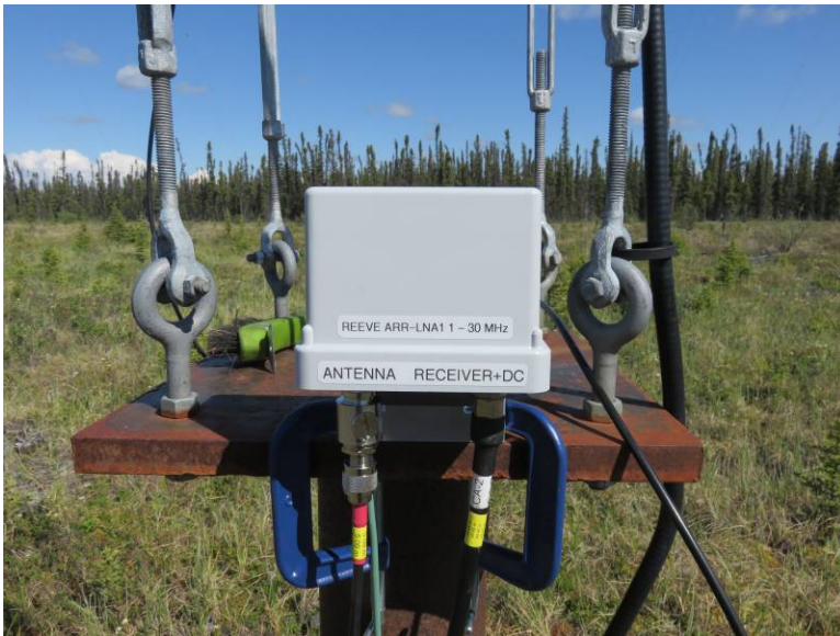
Figure 8 ~ Antenna preamplifier with a gas-tube lightning protector on its input. This photograph was taken just before the coaxial connections were sealed. The amplifier is mounted in a weatherproof enclosure along with type N-F bulkhead connectors and internal RG-316 coaxial cables. C-clamps were used rather than drilling the 1 in thick steel plate on the center piling at the antenna. Note the eye-bolts and turnbuckles in the corners of the plate that support the antenna center structure. Image © 2019 W. Reeve
