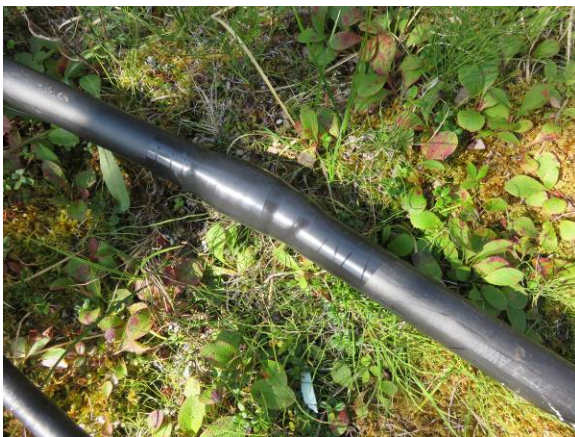
Figure 7 ~ Plastic water pipe used to protect the coaxial cable from rodent damage and tramping by moose. The pipe sections were coupled and taped as shown here. Image © 2019 W. Reeve
