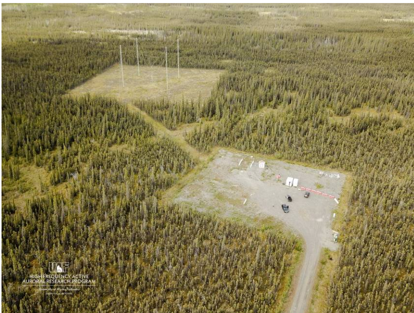
Figure 1 ~ Aerial drone view in June 2019 from about 400 ft altitude (AGL) looking west. The TCI-540 antenna site is in the left-background and the gravel pad for the equipment enclosure is in the foreground. The clearing for the antenna is 160 000 ft 2 (~15 000 m 2 ) and for the pad is 46 000 ft 2 (4300 m 2 ). At one time, the equipment pad included at least two buildings to support the DoD project, but these were demolished before UAF-GI took possession of the facility. The ground-laid coaxial cable transmission line follows a path from the equipment shelter to the southwest the corner of the pad and through the woods directly to the antenna center support described later. Image courtesy of HAARP Program Manager, UAF-GI.
