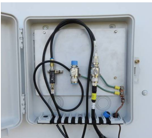
Figure 21 ~ Weatherproof cable entrance protector panel mounted on the back of the equipment enclosure. The panel is a DX Engineering model DXE-UE-2P Utility Enclosure with three protectors mounted on the supplied aluminum plate. The left protector is a Tii Technologies model 212FF75F225-31 that uses type F-F connectors for the Radio JOVE antenna and receiver. The other two protectors, both Citel model P8AX09-N/MF, use a type N-M on the antenna side and N-F on the receiver side. The middle protector is for future connection, and the one on the right connects to the TCI-540 antenna feedline and indoor RF panel. A 6 AWG bare copper conductor bonds the panel to a ground rod. Image © 2019 W. Reeve
