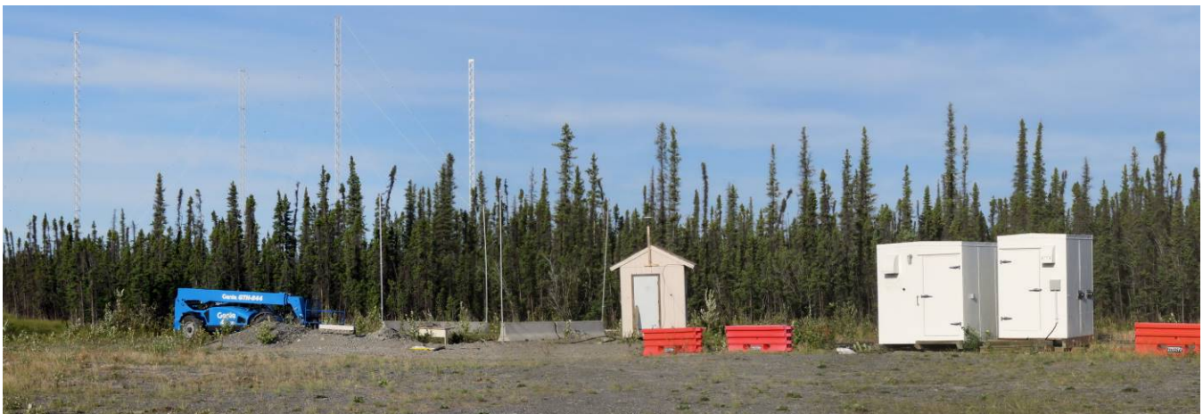
Figure 9 ~ Panorama showing the TCI-540 antenna (towers in the background), Radio JOVE antenna (to the immediate left of the small enclosure with the gable roof) and equipment enclosure for the observatory (larger of two enclosures on the right). The skid-mounted, walk-in, observatory equipment enclosure is 8 x 9 ft (2.4 x 2.7 m) and houses all common equipment and receivers. The two smaller enclosures are not related to the observatory. The blue man-lift on the left was used during erection of the Radio JOVE dual dipole antenna. Image © 2019 W. Reeve
