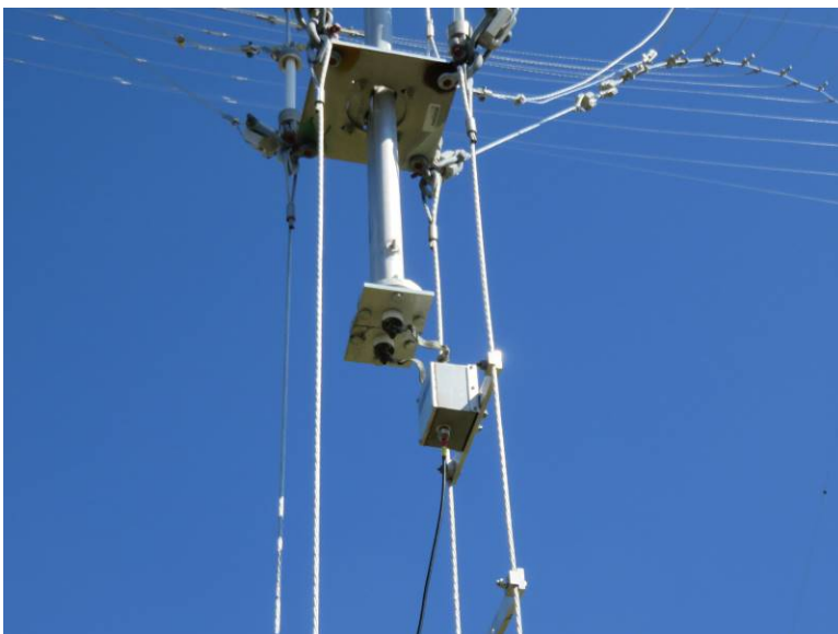
Figure 6 ~ Balun (lower box) and balanced impedance matching and coupling tubes. Flexible braided conductors are visible between the balun and matching tubes. All structural and antenna wire components appear to be made from galvanized steel strand. Image © 2019 W. Reeve
