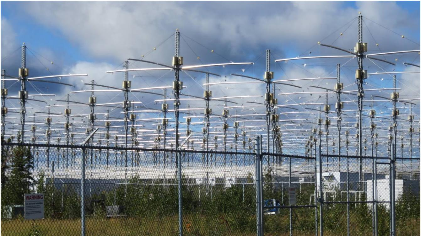
Figure 1 ~ HAARP Ionospheric Research Instrument antenna with collocated transmitters as it appeared on 25 August 2018. With all transmitters active, the IRI is capable of transmitting about 2 GW effective radiated power (ERP) to heat a spot in the ionosphere, but not all were serviceable during the winter campaign. Image © 2018 W. Reeve
