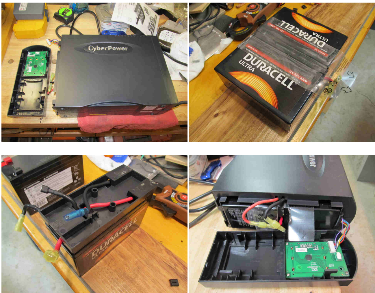
Figure 8 ~ Battery replacement details. (a) Upper-left : The connectorized front panel has been removed and is sitting to the left of the main enclosure. (b) Upper-right : A flexible clear plastic wrapper has adhesive on one side and holds the two batteries to the partition. (c) Lower-left : A hollow plastic partition with a wiring compartment separates the two batteries. One new battery has been connected. The batteries are placed with their terminals at opposite ends of the partition, reducing the chance for a short-circuit. (d) Lower-right : After reassembly of the batteries and reconnection, the front panel is ready for installation. The green printed circuit board on the front panel includes a pushbutton control and display. This
