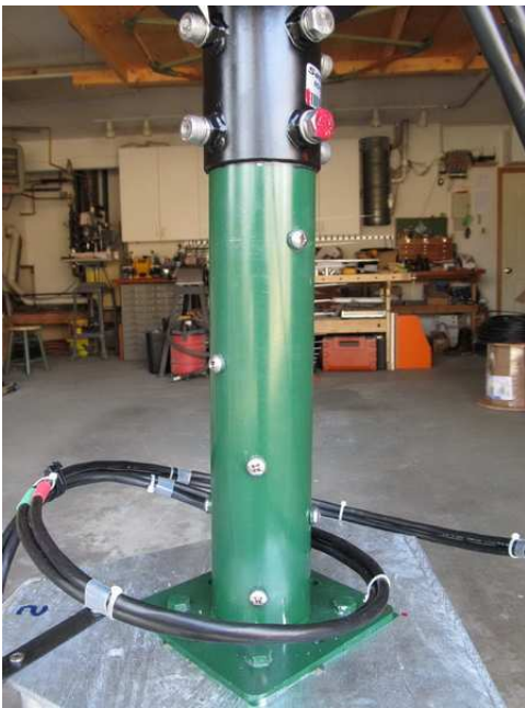
Figure 8 ~ Antenna rotator support mast and mast adapter. The mast adapter at the bottom is steel and the mast is two telescoping sections of aluminum tube. The mast adapter is attached to the tower top plate with 3/8-16 galvanized steel fasteners. The rotator's bottom sleeve (painted black and seen at top of picture) uses eight 10 mm stainless steel fasteners. All other fasteners are 1/4-20 stainless steel. A coil of the two rotator control cables is seen at the bottom. It loops around to the rotator out of the picture. (Image © 2014, W. Reeve)
