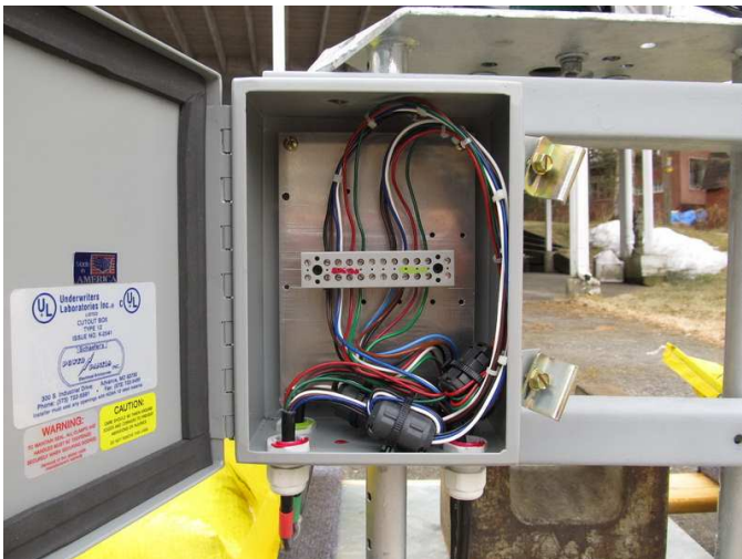
Figure 11 ~ Tower junction box with terminal block to enable termination and paralleling of the rotator control conductors. The box is 8 in high x 6 in wide x 4 in deep and has a rubber gasket on the hinged door. Ferrite beads for noise suppression are seen at bottom of enclosure. All cables are color coded to aid assembly and troubleshooting. (Image © 2014, W. Reeve)
