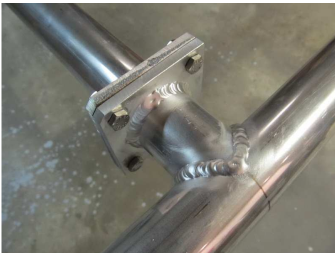
Figure 5 ~ Welds of the horizontal boom, antenna mount and flanges. The bolted flanges allow relatively easy field modifications to the antenna configuration. (Image © 2014, W. Reeve)
