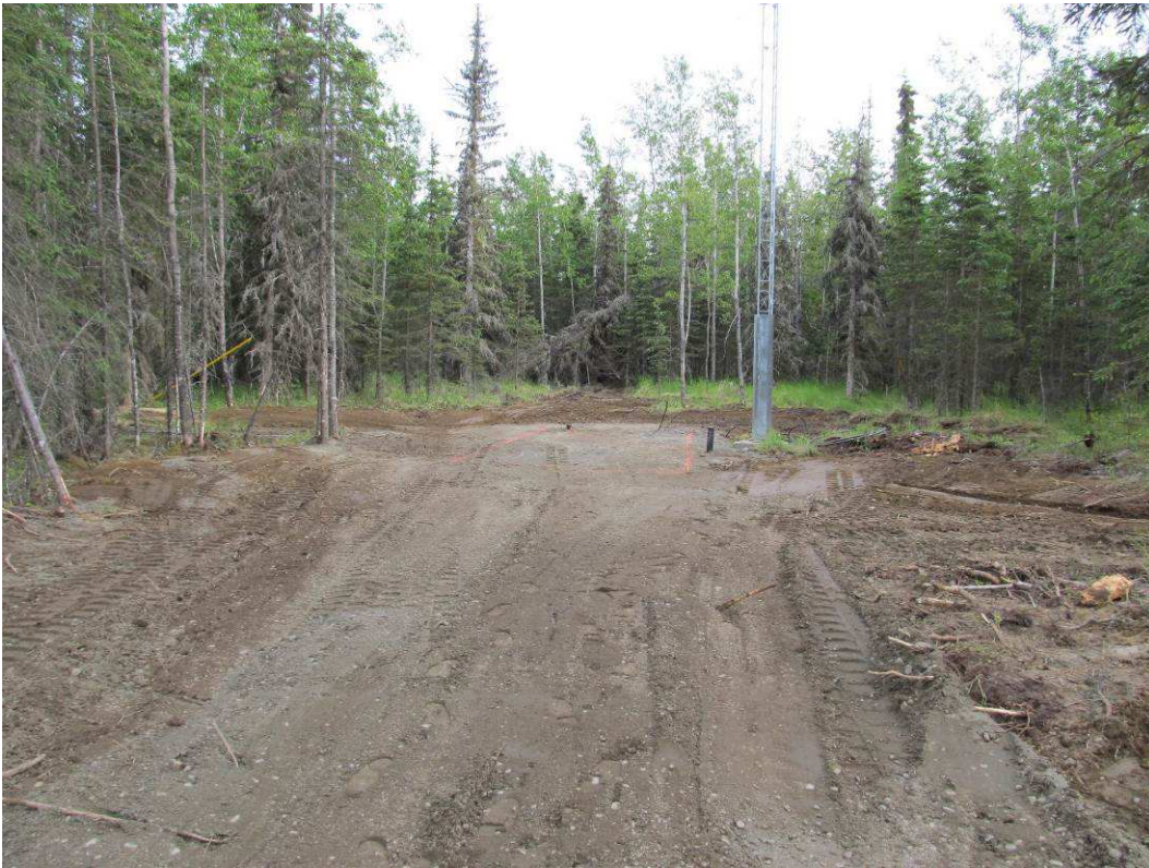
Figure 3 ~ The completed driveway is 100 ft long and 10 ft wide. The tower can be seen in the back at the right. (Image © 2014 W. Reeve)
