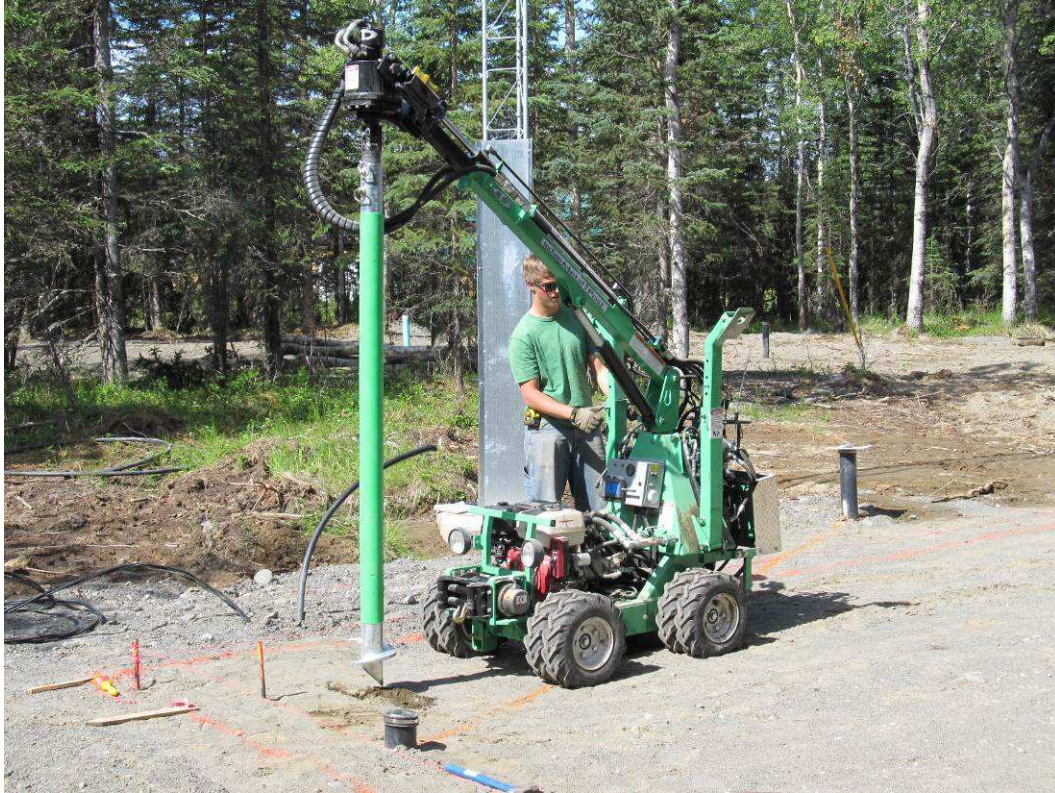
Figure 5 ~ The self-powered post driver (called R2D) was brought to the site in an enclosed trailer hauled behind TMP Alaska’s pickup truck. The machine has local and wireless controls and uses a diesel engine with hydraulic pump. An 8 ft post with helix at the bottom can be seen hanging from the geared hydraulic motor ready for installation. The posts are galvanized steel and covered with green plastic sleeves. The sleeve eliminates frost heaving due to adfreeze of the steel posts and the ground during winter. (Image © 2014 W. Reeve)
