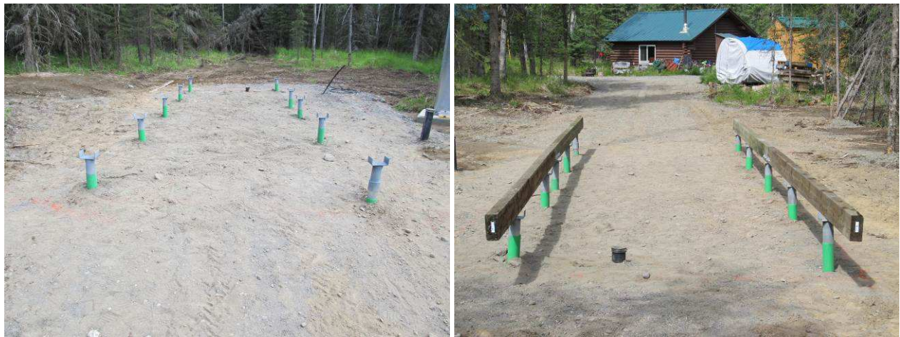
Figure 7 ~ Left : This view looking down the driveway was taken shortly after the ten helix posts were installed. Right : The next day I installed pressure-treated outdoor wood beams for the building to rest on. This view is looking up the driveway toward the original Coho cabin. The foundation was lined up with the driveway so the building could be delivered on a trailer. (Images © 2014 W. Reeve)
