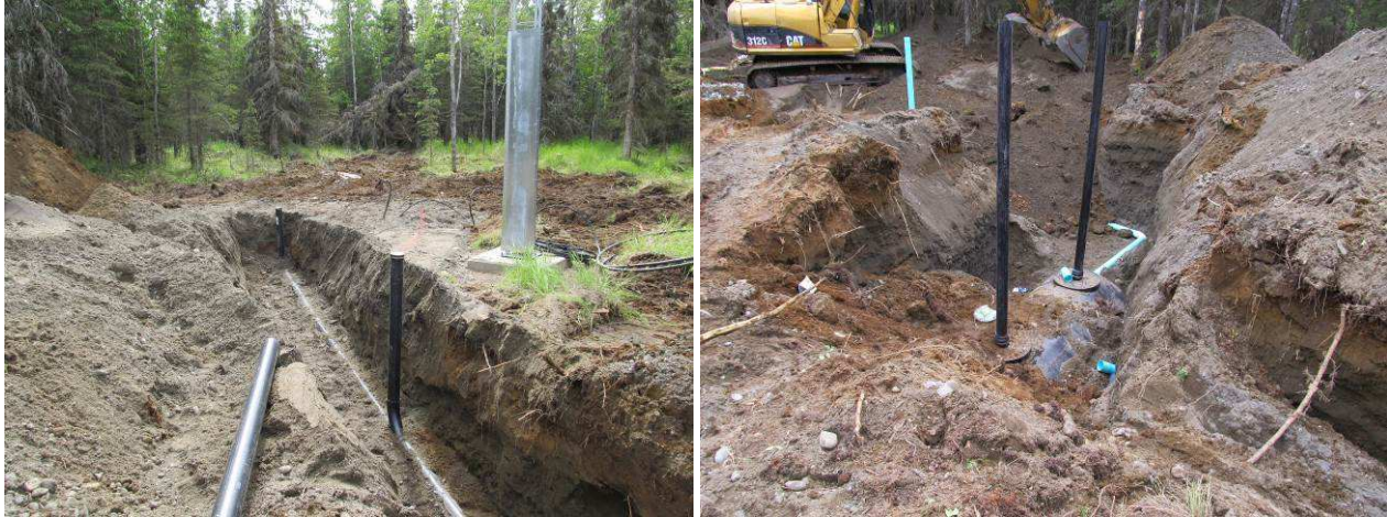
Figure 4 ~ Left : The 4 in sewer line is laid in a trench from the new building location. The vertical pipe in the middle of the picture is a cleanout near the new building. The tower foundation is seen at upper-right. Right : The septic tank is almost completely buried in this picture. The two vertical black pipes are vents and inspection ports. Part of the (turquoise) line to the drain field and a monitor tube can be seen in the background. (Images © 2014 W. Reeve)
