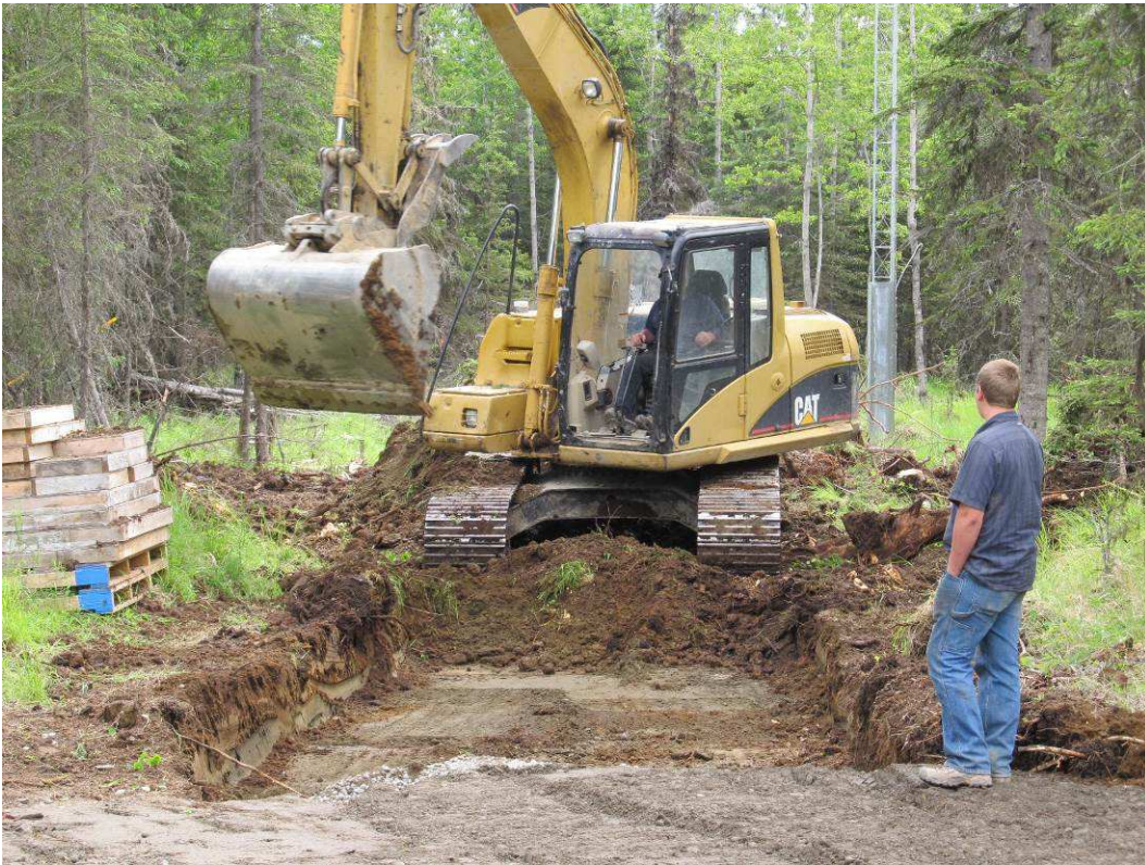
Figure 1 ~ An excavator with a wide bucket removes the top soils from the hard-pan sand and gravel mixture while the contractor's helper looks on. (Image © 2014 W. Reeve)
