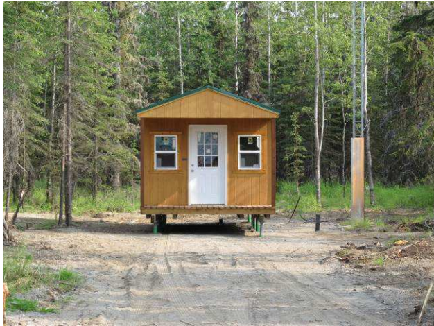
Figure 8 ~ Upper : Observatory building resting on its foundation the day after delivery. The stairs have not yet been built but all other exterior work is completed. The green metal roofing sheds snow very easily, so an ice bridge will be built between the tower and building cable entrance to protect the coaxial and rotor control cables to the tower. Lower-left : View of the observatory building from the end of the driveway. The tower can be seen on the right. Lower-right : Inside view of unfinished building looking toward the front. The roof is made from built-up trusses and the cavities between floor joists are sealed and insulated. The usable interior floor space is approximately 250 ft 2 and walls are 8 ft high (Images © 2014 W. Reeve)
