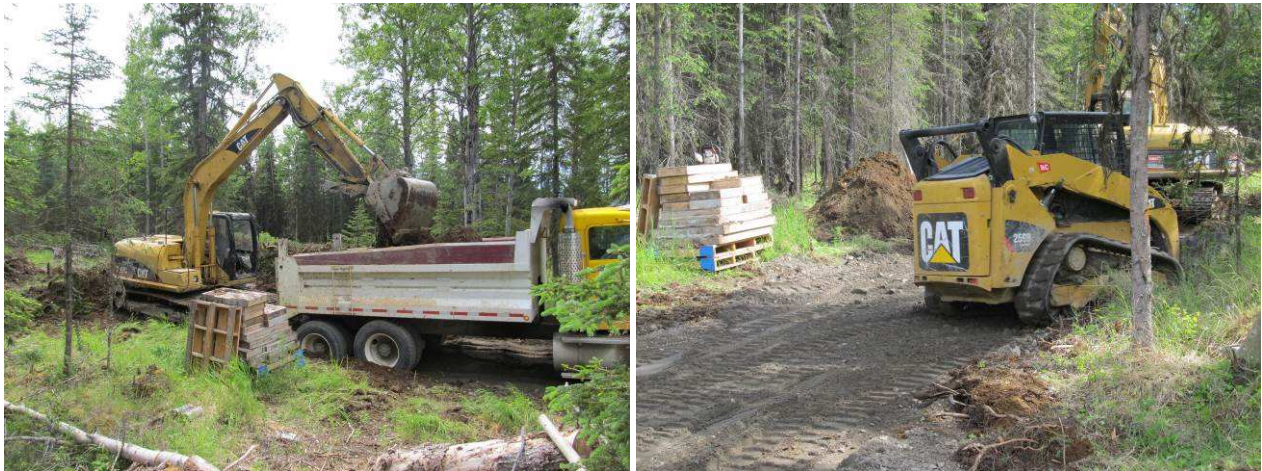
Figure 2 ~ Left : After dumping a load of sand and gravel backfill, the dump truck is loaded with the roots and top soils to be disposed of. Right : A small tracked front-end loader spreads, compacts and levels the backfill in the driveway. (Images © 2014 W. Reeve)
