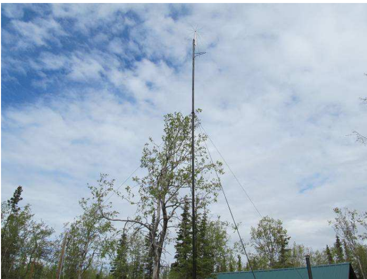
Figure 10 ~ Mast raised and in-use. Rope guys angled away from the mast can be seen approximately 2 m below top of mast. Discone antenna and relief loop in coaxial cable are barely visible.
