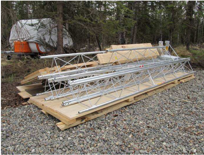
Figure 11 ~ Tower sections resting on the crate material in which they were shipped.
