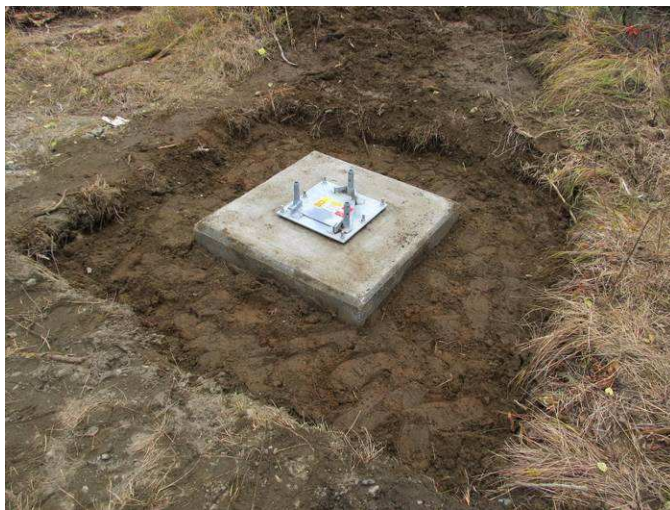
Figure 10 ~ Holes were backfilled using the native soil and the “Armstrong Method”. The base is ready to accept the first tower section.
