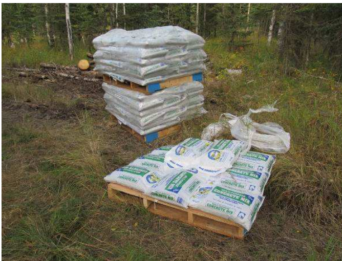
Figure 6 ~ A total of 118 out of 130 bags of concrete/aggregate mix, delivered on wood pallets, were used in the tower base and anchors.
