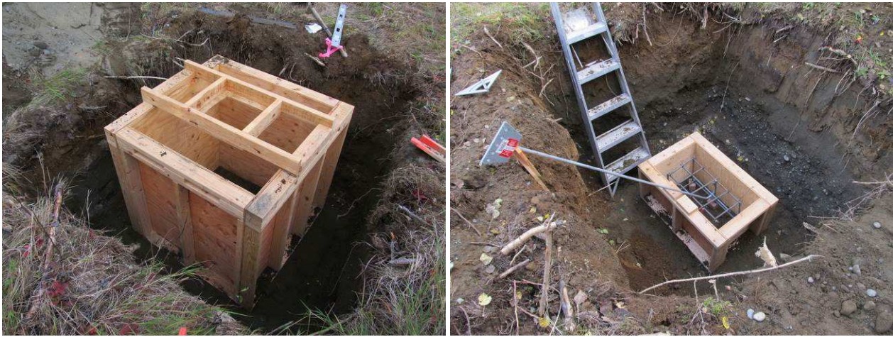
Figure 5 ~ Upper-left : The pre-built wood forms were easy to assemble in-place with screws to hold the four sides together. Upper-right : Reinforcing steel was cut to length by a supplier in Anchorage. Lower-left : The base form has been placed and leveled. The H-frame at top is a template that holds the tower base plate in position while the concrete cures; fixed wood blocks hold the H-frame in alignment. The reinforcing steel has not yet been placed. Lower-right : One of the anchor forms with the reinforcing steel in-place. The anchor rod projects up and out of the form to the left of the image. The lower end of the anchor rod has a hook to increase its pull-out resistance. The hole for each anchor is 4 ft deep.
