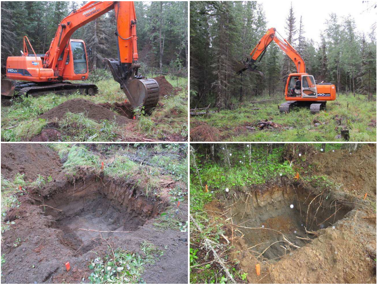
Figure 4 ~ Upper-left and -right : The excavator eliminated a lot of hard, back-breaking work. It was well equipped with a large bucket, claw on the bucket for grabbing and moving trees and roots and a blade at the front for scraping peat. I asked the operator to pile the different soils separately so I could later backfill with the same soil at depth. Lower-left and -right : Base and anchor locations ready for the concrete forms. The intact layout stakes seen in each corner attest to the operator's accurate digging skills. The three soil layers are clearly visible in these images, in order peat, clay, and gravel.
