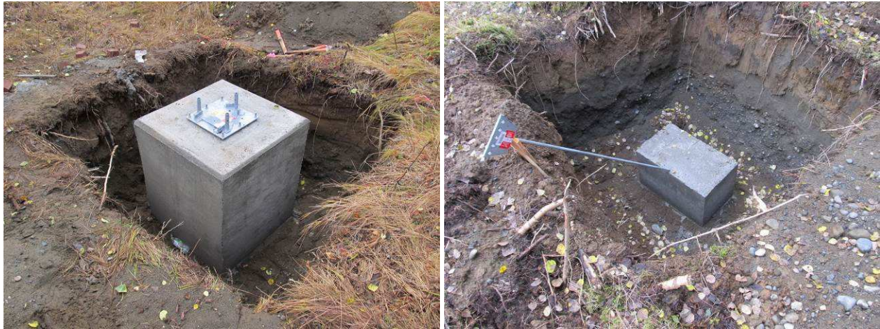
Figure 9 ~ Wood forms have been removed and holes are ready for backfill. Left : The base was poured with a 1 in chamfer around the top, something not seen on many small tower bases. This view also shows the tower base plate bolted in position. The base weighs about 4725 lb. Right : One of the anchors ready for burial. Each anchor weighs about 844 lb.
