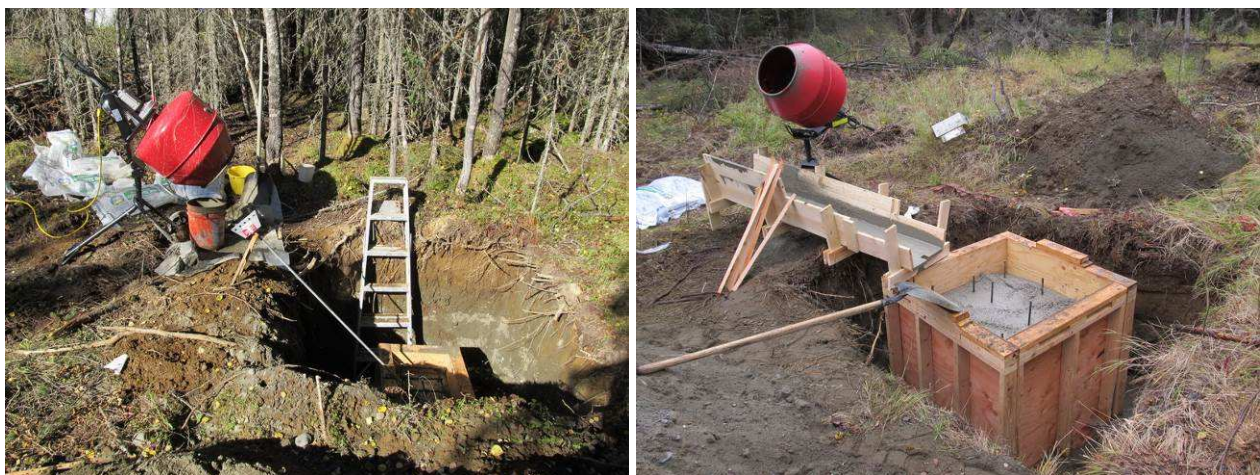
Figure 8 ~ Left : The cement mixer was placed at each anchor next to the hole, and a 5 gal bucket was used to transfer about 60 lb of mixed concrete at a time. After filling the bucket it was placed on the edge of the hole, lifted down into the hole
