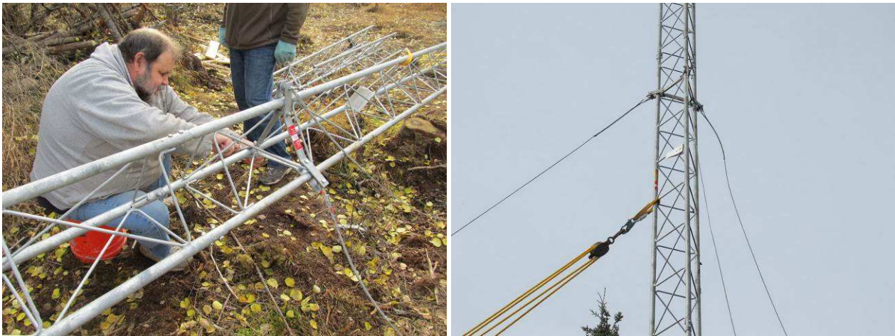
Figure 5 ~ Left : Guy strands were pre-installed on the lower guy brackets by two helpers who knew what they were doing. Right : Lower guy bracket and block-and-tackle immediately after raising the four tower sections. The guy wire to left is under tension while it is being installed, and the other two are still slack while awaiting installation. (Images © 2014, W. Reeve)
