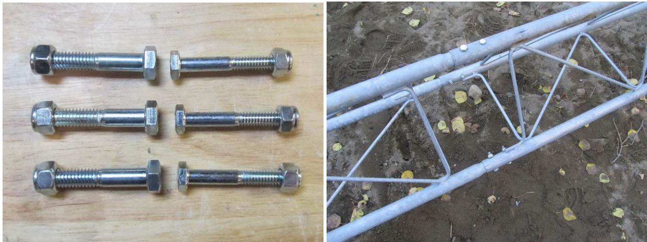
Figure 10 ~ Left : Each tower section leg is held to the section below it with two bolts, 1/4 in and 5/16 in diameter, and nylon lock nuts. Right : Tower bolts before the four tower sections are raised. (Images © 2014, W. Reeve)
