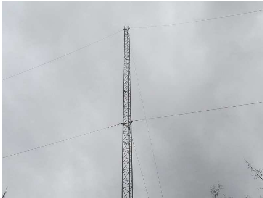
Figure 12 ~ Upper tower sections showing the guy brackets and wires. (Image © 2014, W. Reeve)
