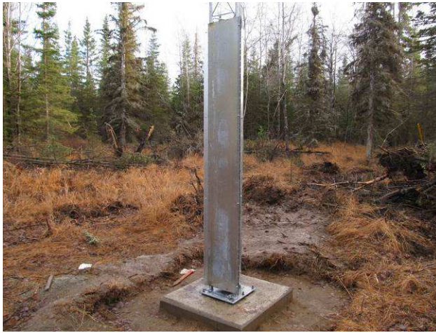
Figure 14 ~ Left : Anti-climb panels are 8 ft long. The tower cannot be climbed without using a ladder or removing the panels. Right : Work platform can be temporarily installed at almost any location on the tower. The work platform at first seemed to fit like socks on a rooster but once figured out it easily clips on. (Image on left © 2014, W. Reeve, source of image on right unknown)
