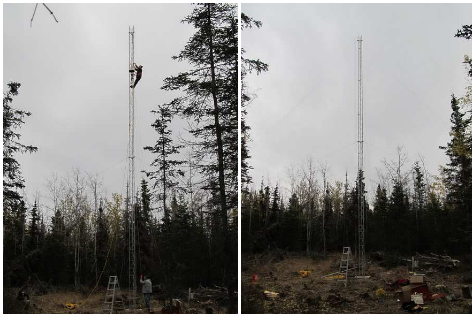
Figure 11 ~ Left : Guiding the last tower section into place. Right : Tower assembly at full height while guy wires, barely visible against the overcast sky, are being tightened. (Images © 2014, W. Reeve)
