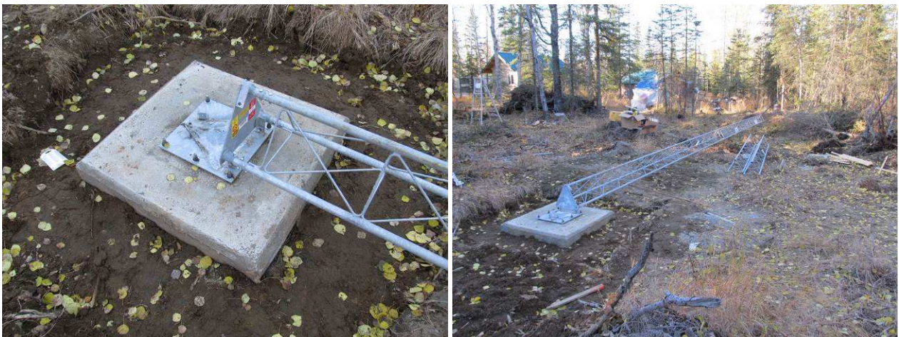
Figure 4 ~ Left : The hinged base plate is held with six J-bolts embedded in the concrete. The two hinges on the right side of the base are installed with 1/2 in fasteners. After the tower is rotated to vertical, the base is held closed by two brackets
