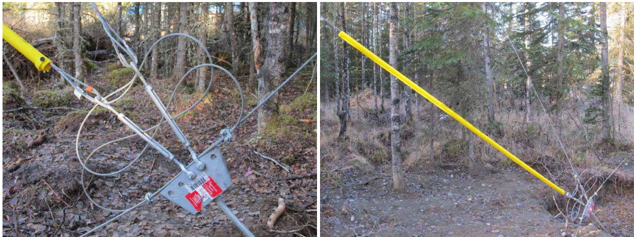
Figure 13 ~ Guy anchor and guy strand. Left : Turnbuckles at the anchor rod plate are prevented from turning by looping the guy wire tails through them and then clamping with guy clips. Right : Yellow guy markers improve visibility of the almost invisible guy strand. (Images © 2014, W. Reeve)
