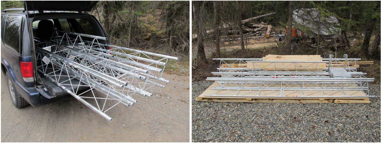
Figure 3 ~ Tower sections were moved a couple hundred feet in the back of my SUV (left) and restacked for the winter (right). The hot-dipped galvanizing used on all steel components was very shiny when delivered but it oxidized and dulled over the winter, as I expected. (Images © 2014, W. Reeve)
