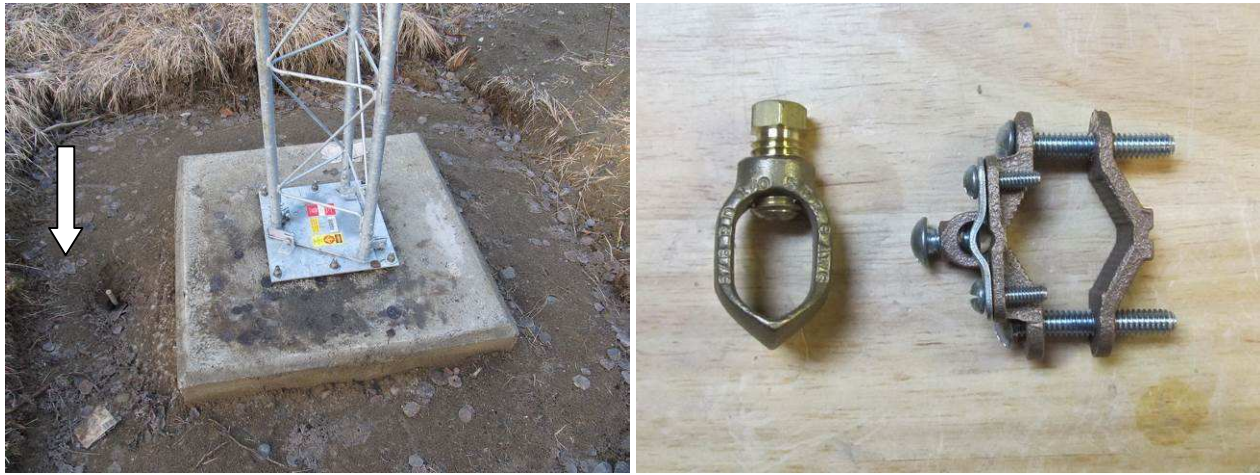
Figure 15 ~ Left : The tip of the ground rod (arrow) for the tower base is visible poking out of the quickly freezing ground. In spring 2014, it will be cleaned with emery cloth and painted with anti-oxidant before attaching the ground rod clamp and 6 AWG bonding conductor. The closest tower leg will be similarly prepared for a bonding clamp. Right : The ground rod clamp (left) and tower bonding clamp (right) ready for installation. (Images © 2014, W. Reeve)
