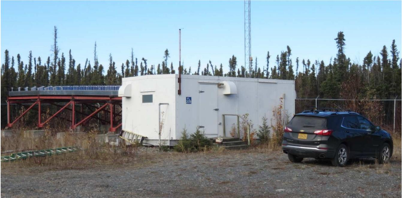
Figure 3 ~ MUIR equipment enclosure and associated radar antenna array (left-background). All electronics for the Callisto-LWA installation were placed in the enclosure at the end of September. A protected coaxial cable entrance facility was installed on the back of the enclosure (not visible in this picture). This picture was taken the day before the weather station and lightning sensor was installed on the enclosure. Image © 2021 W. Reeve
