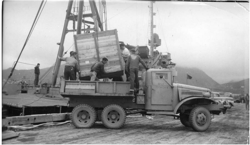
Loading crates of eclipse expedition equipment onto truck, Attu, Alaska
