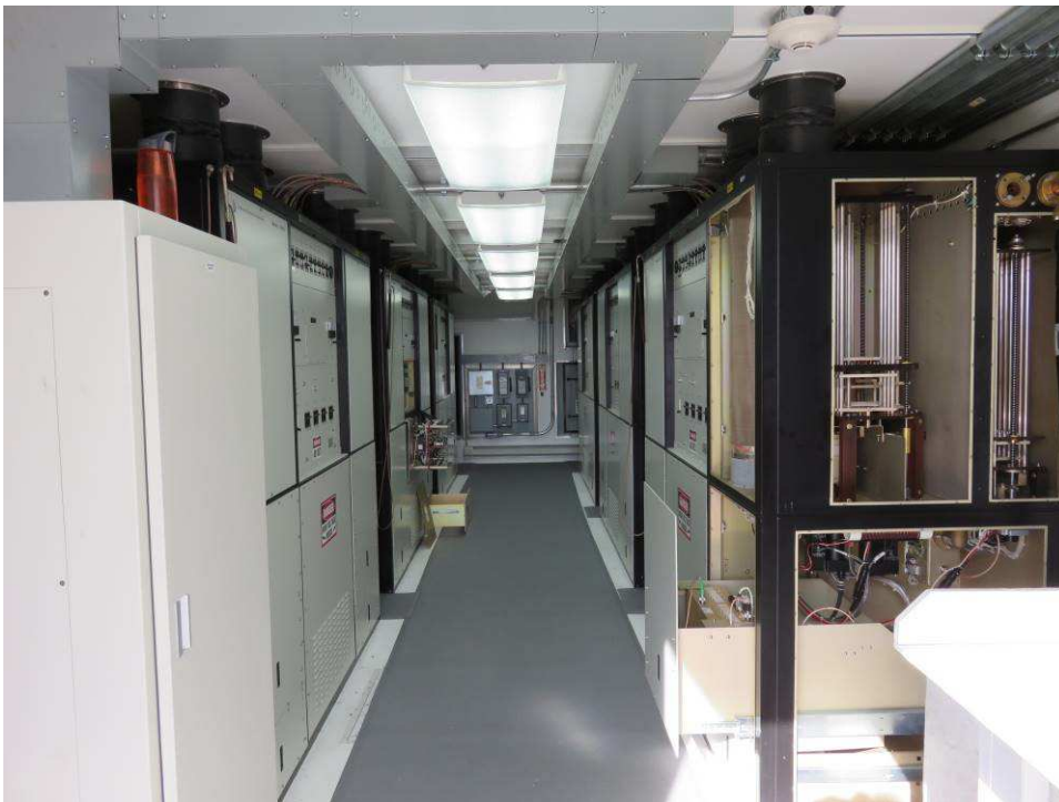
Figure 6 ~ Interior view of a typical transmitter enclosure. A central aisle provides front access to equipment cabinets on either side. On the near-right, one of the transmitter cabinets has been opened for examination. I believe the exposed components in the two upper compartments are motorized tuning inductors or capacitors (or both). Image © 2016 W. Reeve
