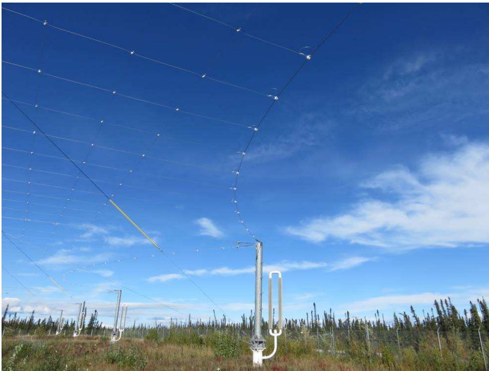
Figure 19 ~ View of one edge of the ground plane against a blue sky. The ground plane extends from the center to left side of the image. It covers a larger area than the antennas. The thermal piles shown here provide support for the ground plane and also are anchors for the antenna support structures. Image © 2016 W. Reeve
