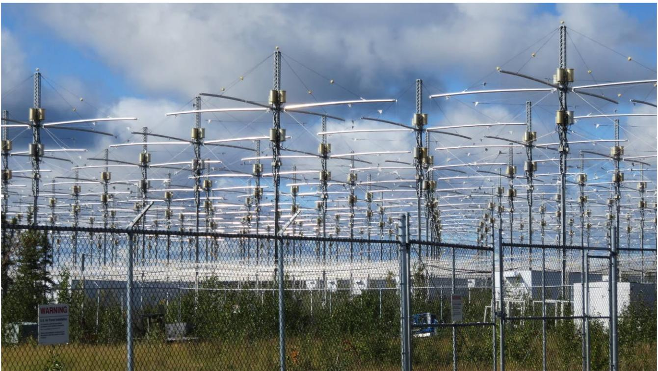
Figure 1 ~ HAARP Ionospheric Research Instrument antenna with collocated transmitters as it appeared on 25 August 2018. It consists of 180 crossed-dipole antennas in a 12 x 15 array but not all antennas are serviceable as of this writing (late 2018) and not all antennas are used in every experiment. The white structures almost hidden by foliage are the transmitter enclosures. Part of the surrounding fence is in the foreground. Image © 2018 W. Reeve
