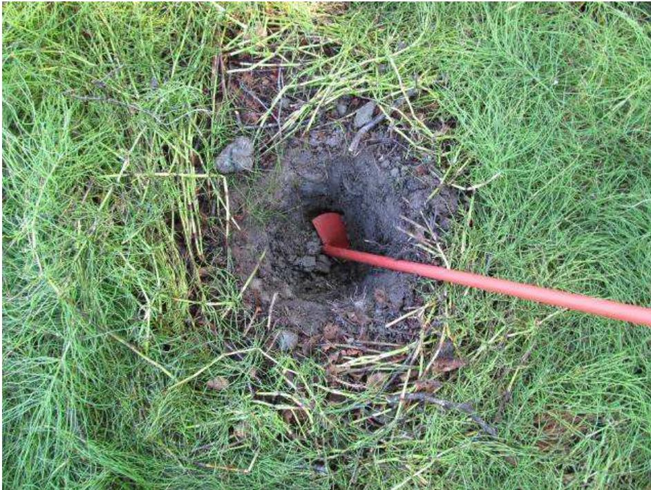
3. Start the anchor by hand, screwing it into the soil until it “bites” and starts pulling itself in. In stiff soils, some downward pressure will be needed.
