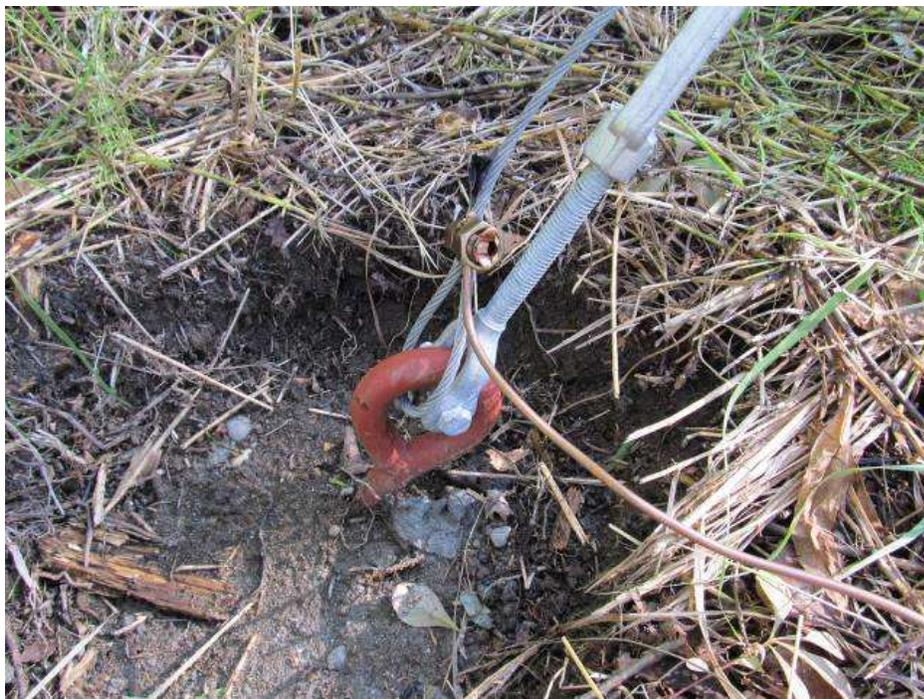
13. Guy wire bonding detail shows the 6 AWG bare copper earth electrode conductor. This picture also shows the guy strand looped through the anchor eye and back up where it is clamped. Bury the earth electrode conductor so that it does not become a tripping hazard.
