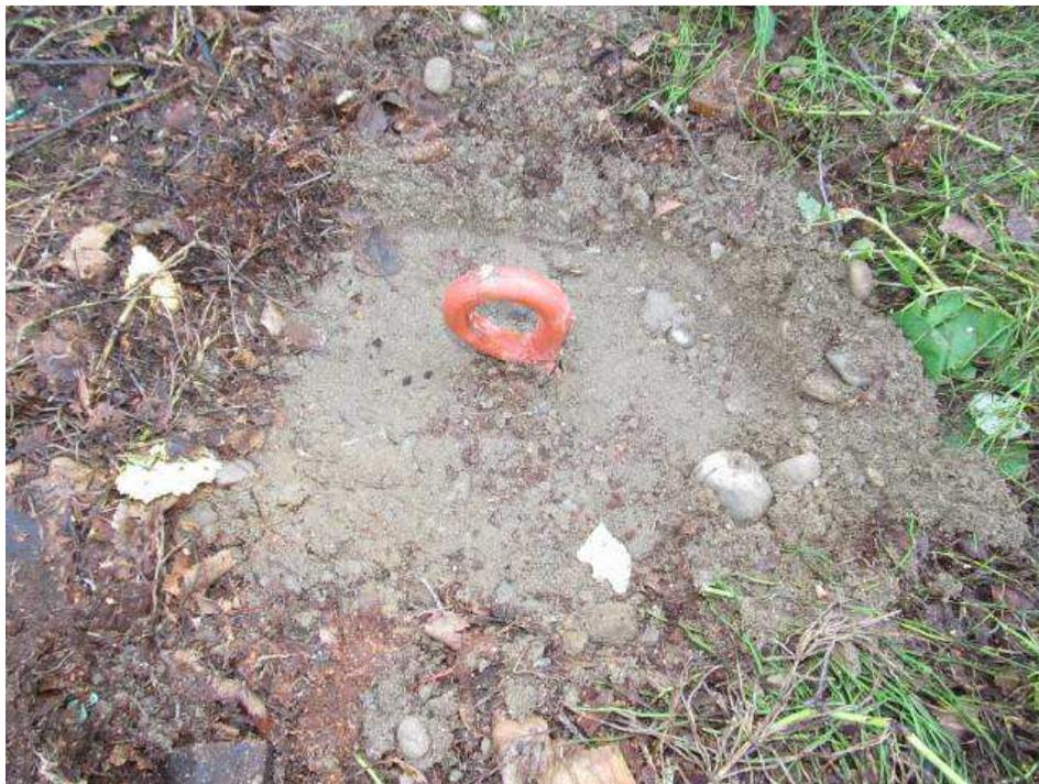
7. Complete the anchor installation by backfilling the starter hole and tamping the soil.
