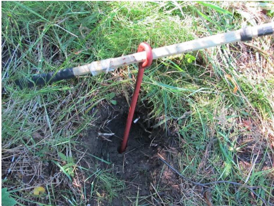
5. Stop every once in a while to rest and admire your hard work. The axe handle used to turn the anchor is shown in-place in the anchor eye.
