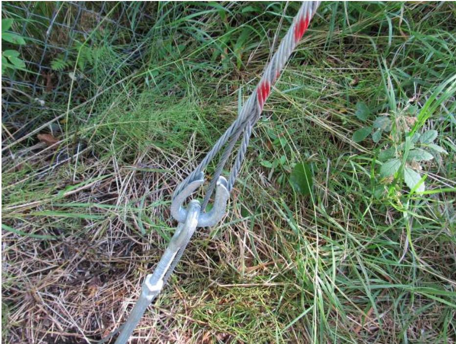
9. Another view of the guy grip showing the thimble and the upper end of a turnbuckle. The thimble protects the wire rope from chafing in the turnbuckle eye. The guy wire extends through the guy grip (see next step).
