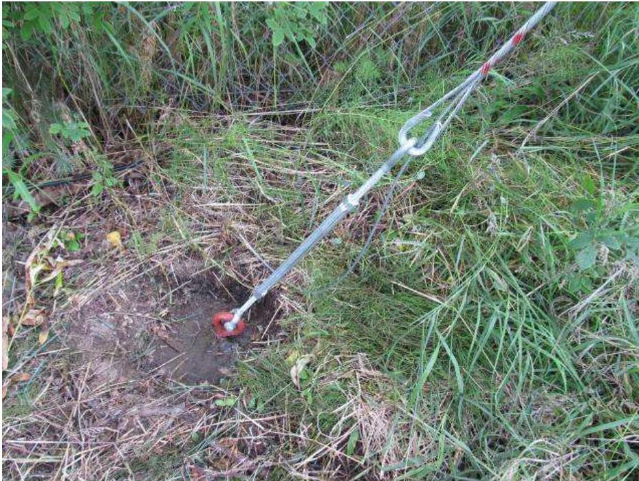
11. Another view of the anchor eye, turnbuckle, thimble, guy grip, and guy wire. After all guys are installed they are tensioned by adjusting the turnbuckle.
